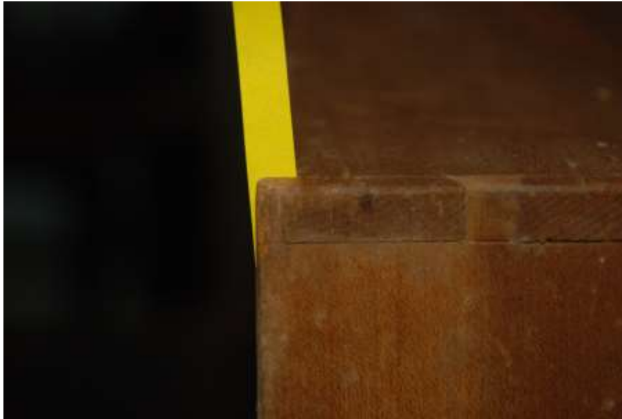
Figure 7. Rear dovetail of the Christopher Townsend drawer showing the tail is tapered at the base of the inner face while the tip of the tail is straight and untapered.
